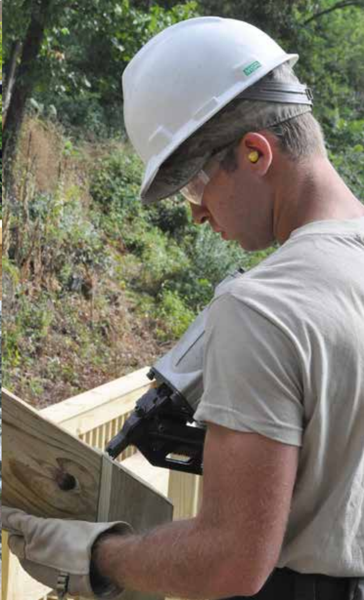
Tech. Sgt. David Morrison, a Civil Engineer structural engineer, uses a nail gun to secure a piece of treated lumber to the new staircase leading from the Veteran's Park to the riverside.
